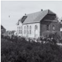
Station Moorslede (PV2013_162-01)
